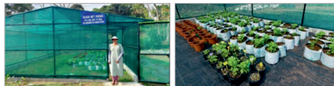
Exterior and interior view of newly built shade house
