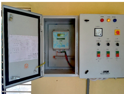
Drip fertigation sensor control panel
