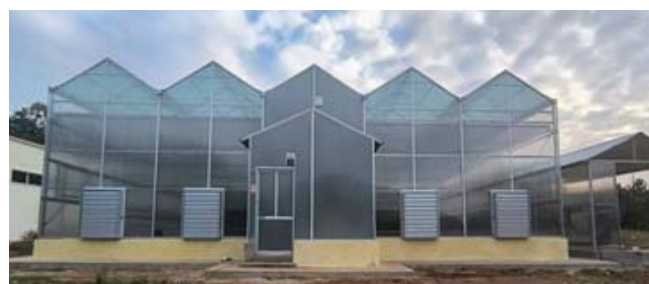
Fig. 93. View of the aeroponics facility under construction.
