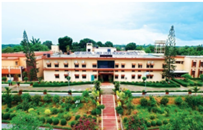
ICAR-CTCRI, Headquarters, Thiruvananthapuram (48.19 ha)
